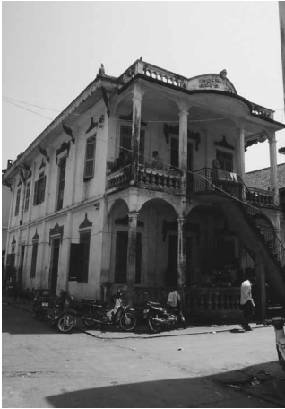
Photo 2 Kot built by Mr. LH in Vatt Unnalaom
